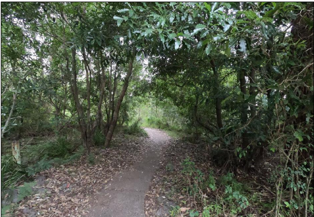
Figure 16. Typical section of existing concrete path through coastal terrestrial vegetation; to be replaced with 1800mm wide new concrete path.
