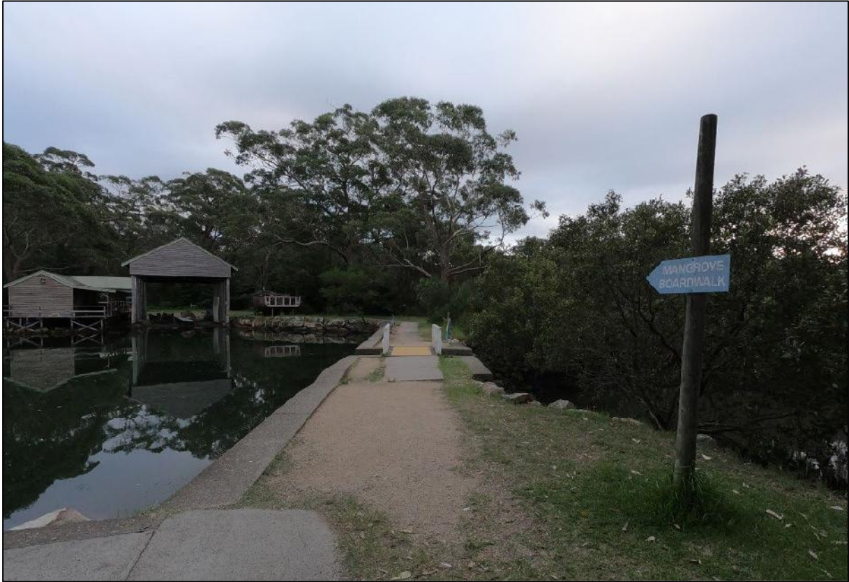
Figure 15. Existing pathway and bridge over sluice structure, to be replaced and widened to 1800mm.
