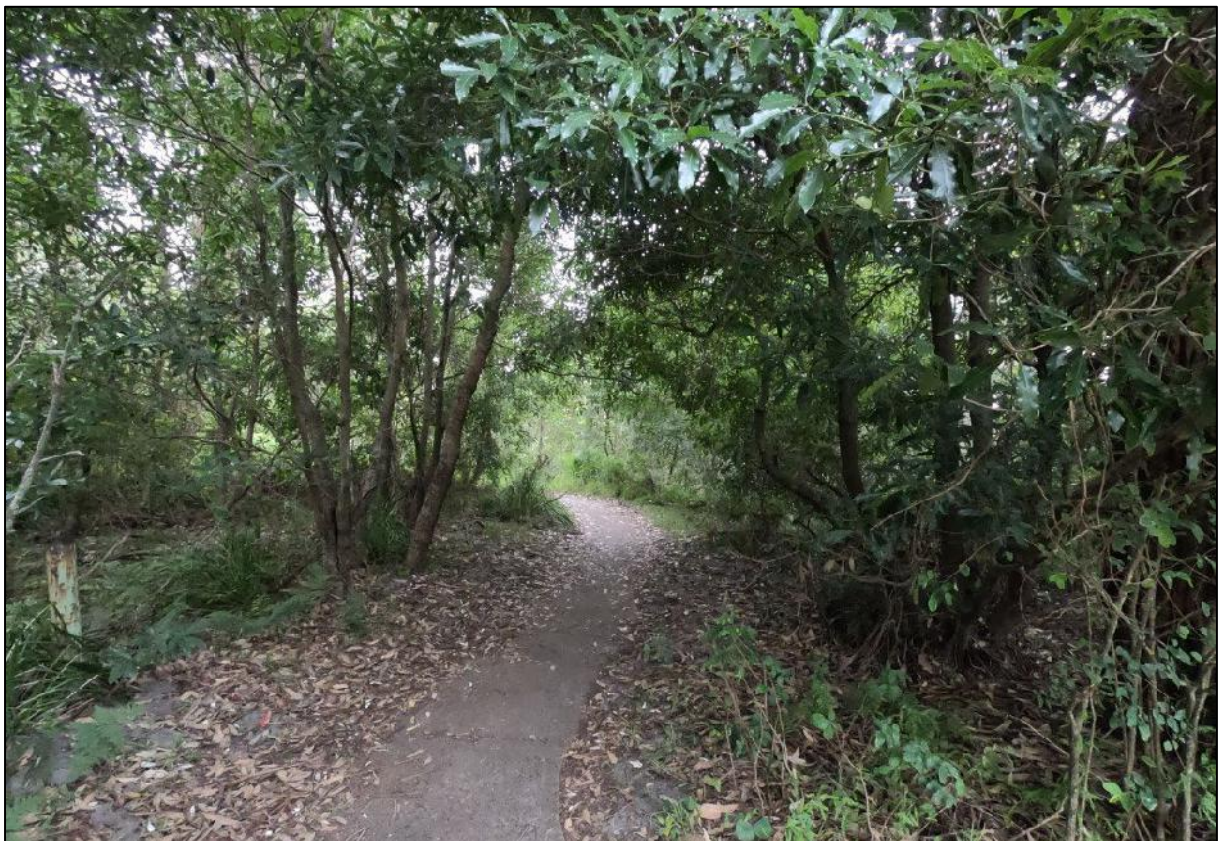
Figure 2. Typical section of existing concrete path through coastal sand forest; to be replaced with 1800mm wide new concrete path.
